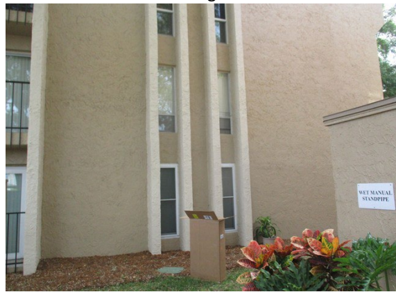
38 Left Side of Building
