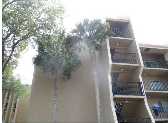
76 Front of Building
