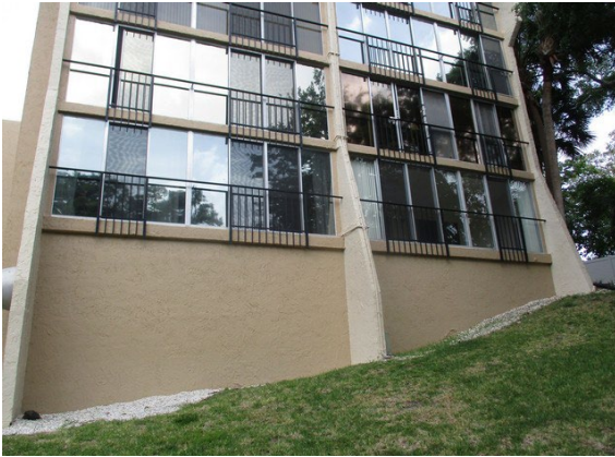
43 Left Side of Building
