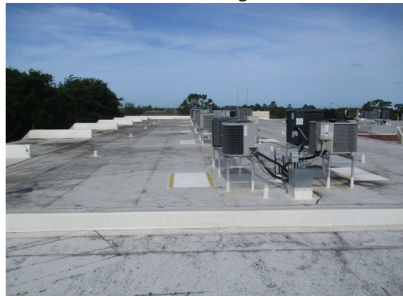
54 Roof Overview Building B
