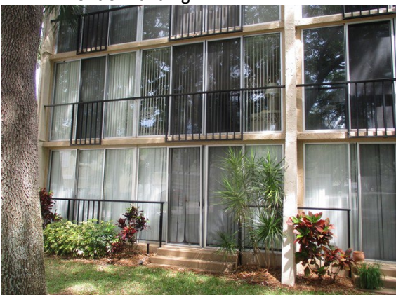
79 Right Side of Building
