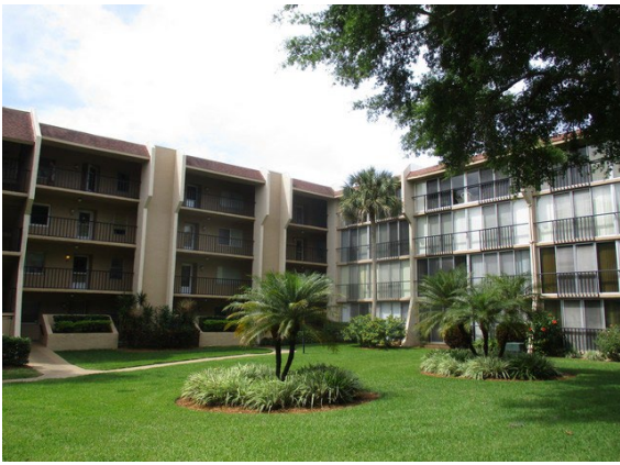
49 Rear of Building B
