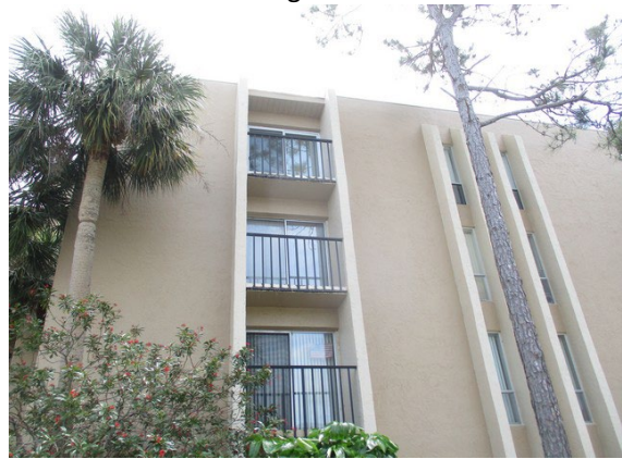
78 Front of Building
