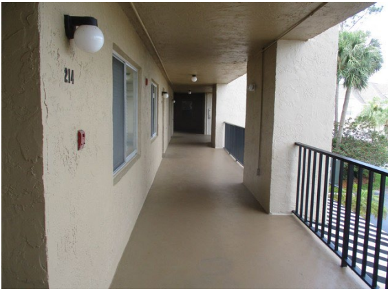
73 2nd Floor Walkway Overview
