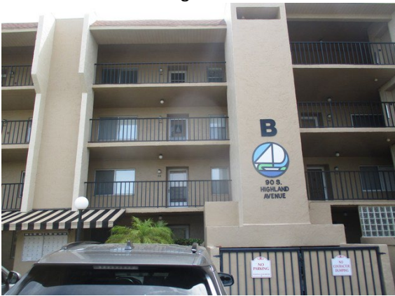
77 Front of Building
