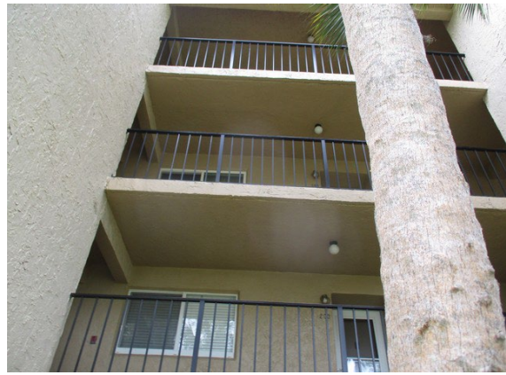
34 Front of Building
