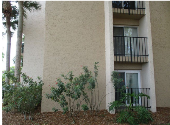
36 Left Side of Building
