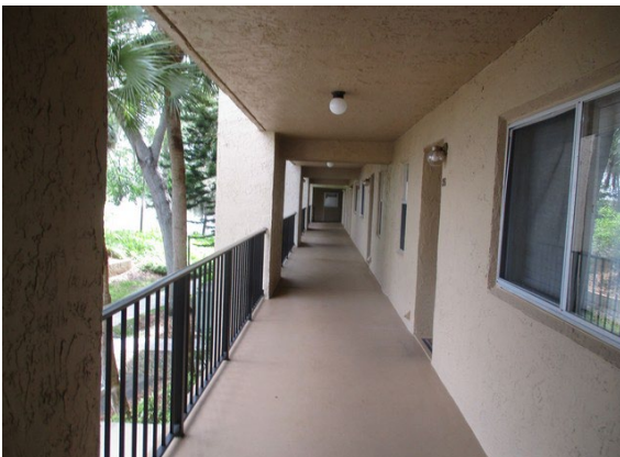
31 2nd Floor Walkway Overview
