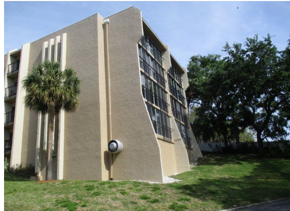
4 Left Side of Building A
