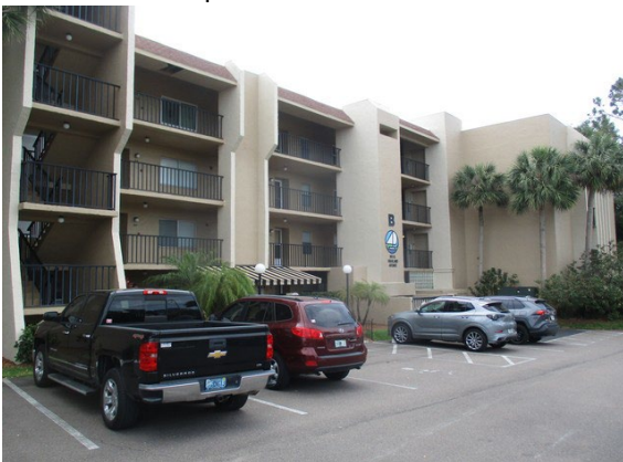
47 Front of Building B
