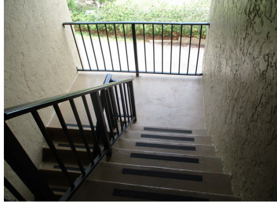
28 Center Stairwell Overview
