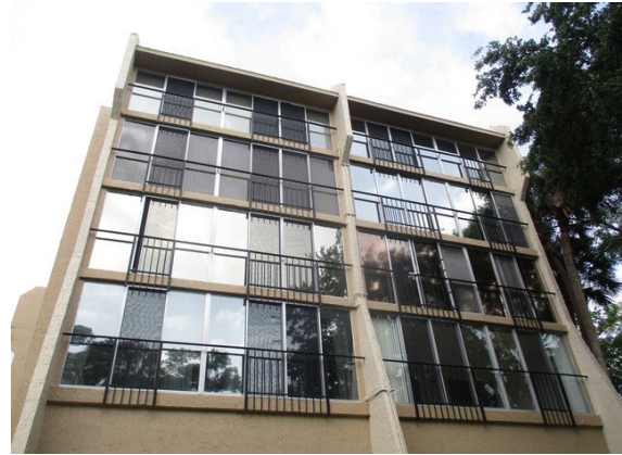
44 Left Side of Building
