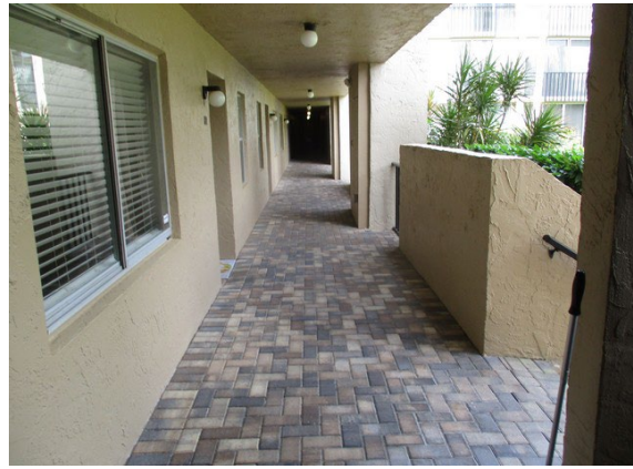
74 1st Floor Walkway Overview
