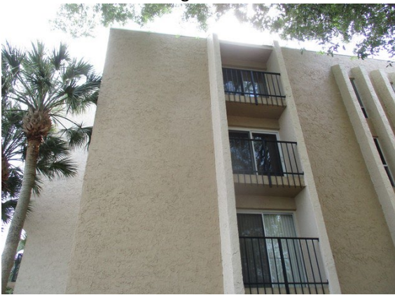
37 Left Side of Building
