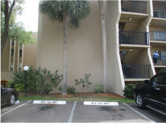
75 Front of Building
