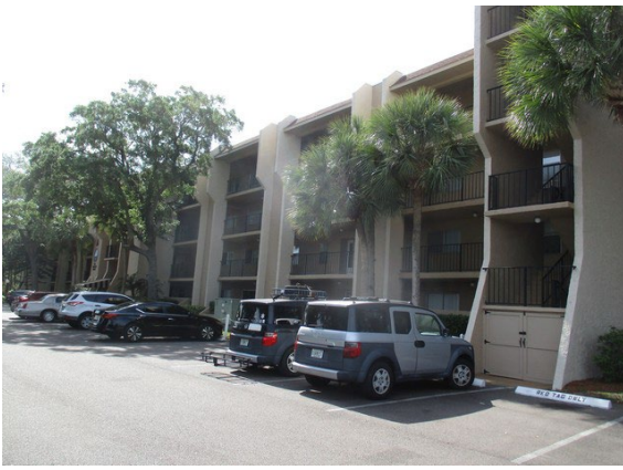
1 Front of Building A
