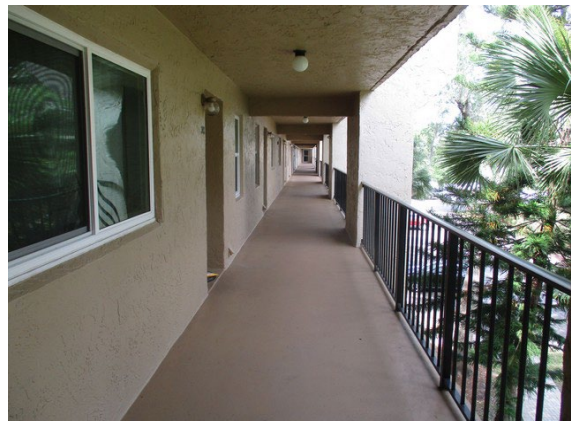
30 3rd Floor Walkway Overview
