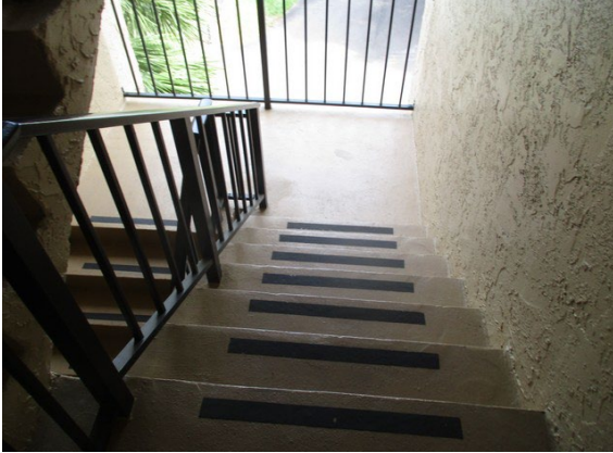
27 Right Stairwell Overview
