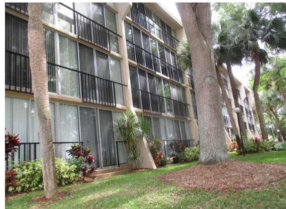
48 Right Side of Building B
