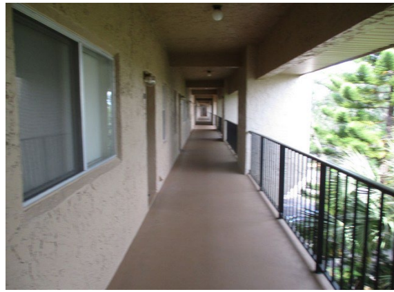
26 4th Floor Walkway Overview
