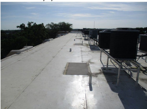
7 Building A Roof Overview
