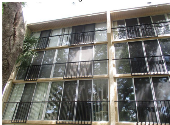
80 Right Side of Building
