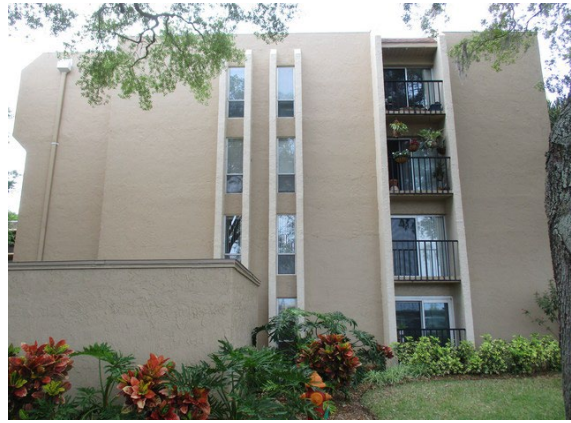
50 Left Side of Building B
