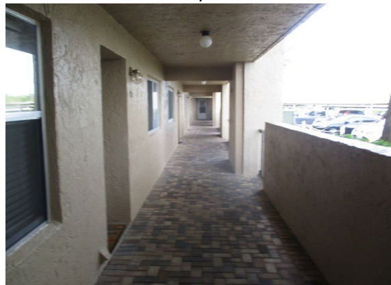
32 1st Floor Walkway Overview
