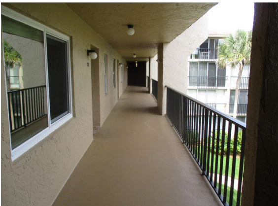
71 3rd Floor Walkway Overview
