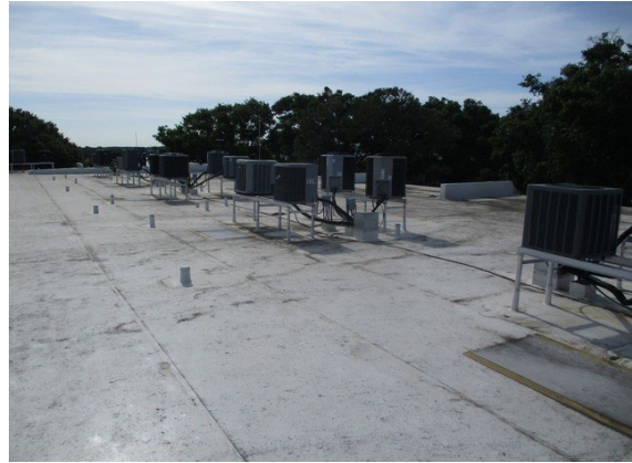
52 Roof Overview Building B
