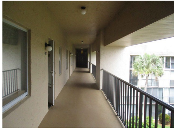
68 4th Floor Walkway Overview
