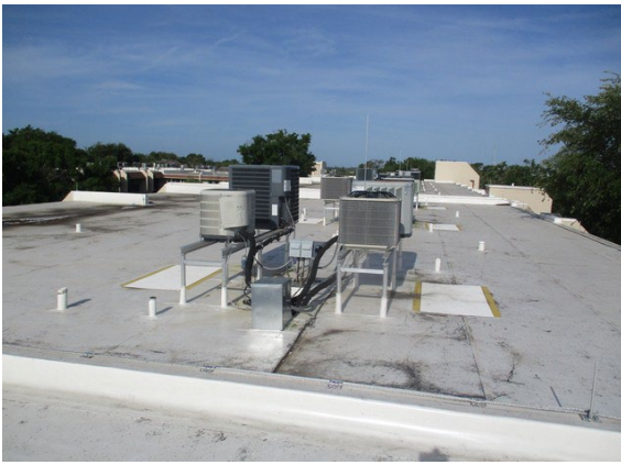
9 Building A Roof Overview
