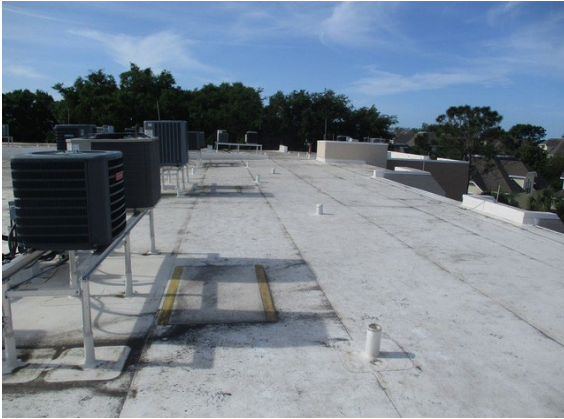
51 Roof Overview Building B
