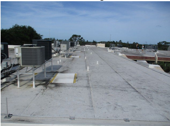
53 Roof Overview Building B
