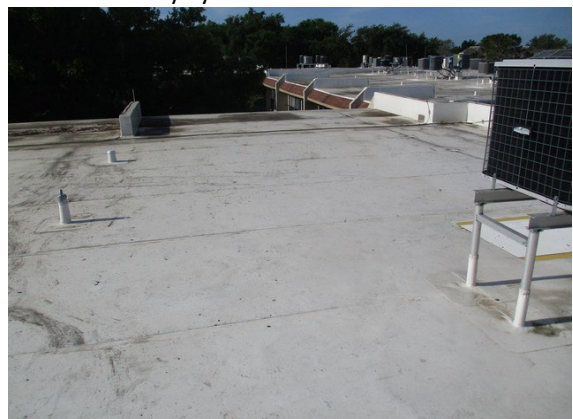
8 Building A Roof Overview
