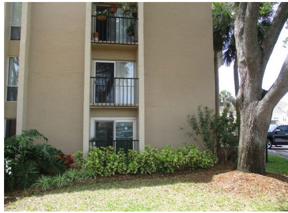
34 Left Side of Building
