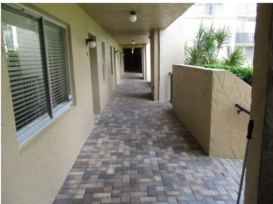
21 1st Floor Walkway Overview
