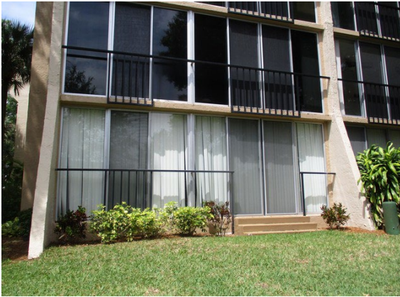
27 Right Side of Building
