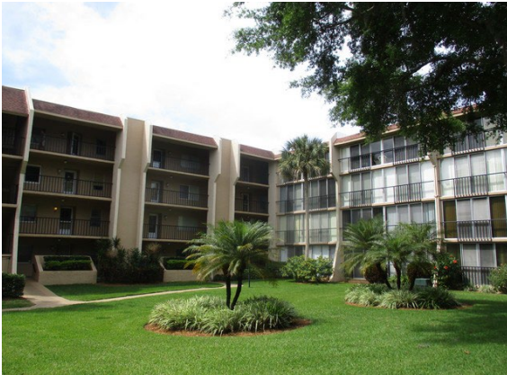
3 Rear of Building B
