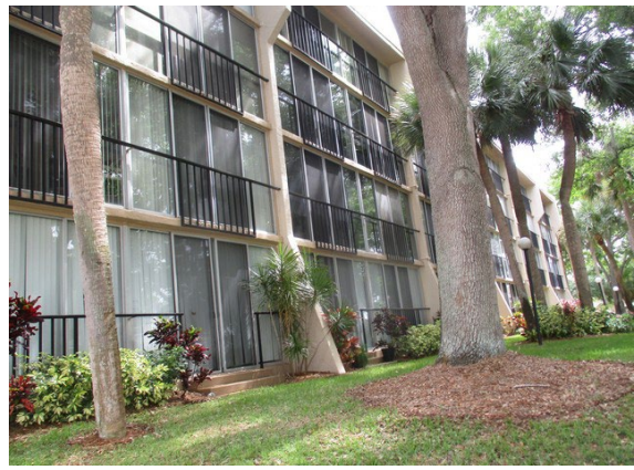
2 Right Side of Building B
