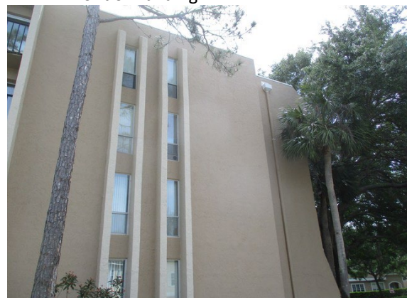
24 Front of Building
