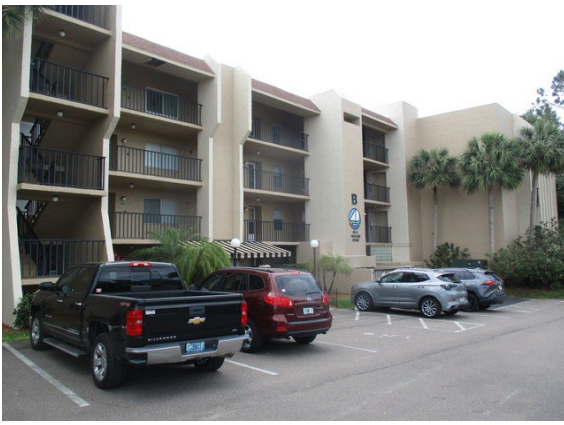
1 Front of Building B
