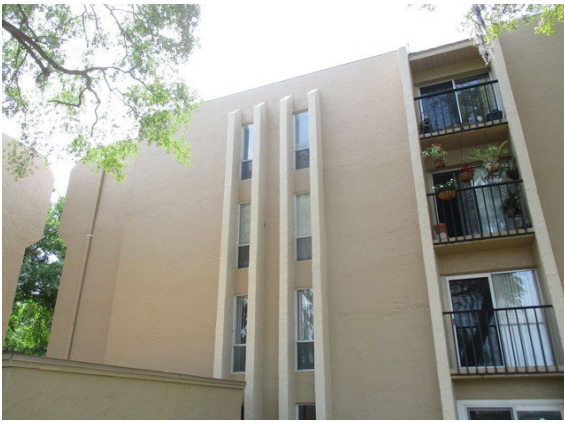
33 Left Side of Building
