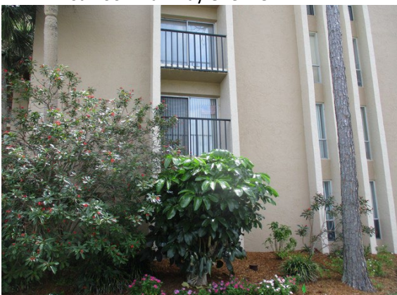
23 Front of Building
