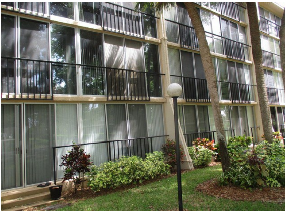
25 Right Side of Building
