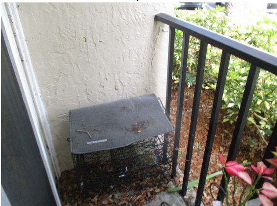
13 Unit #113 Ground Floor Balcony/Porch
