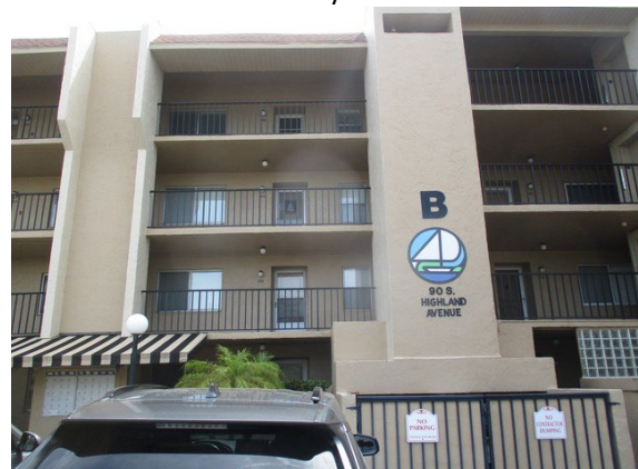
22 Front of Building
