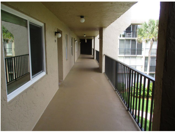
17 3rd Floor Walkway Overview
