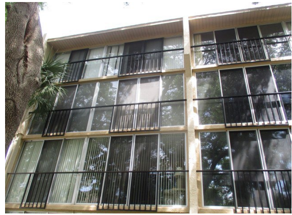
26 Right Side of Building
