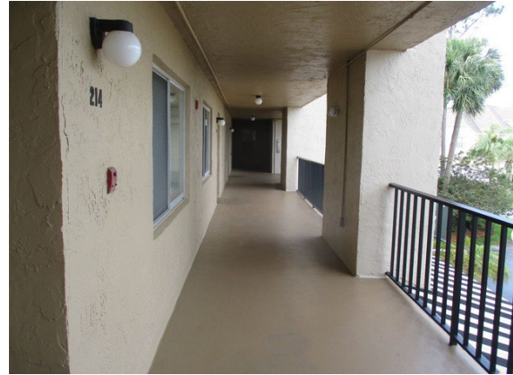
20 2nd Floor Walkway
