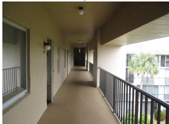
14 4th Floor Walkway Overview
