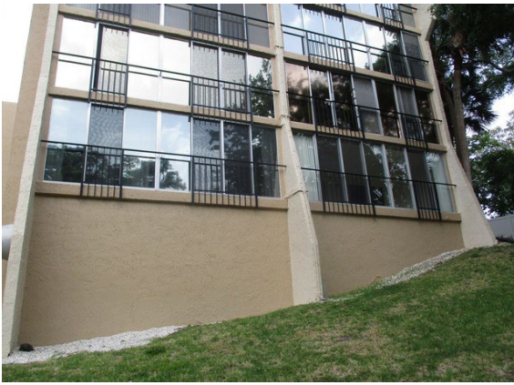
33 Left Side of Building
