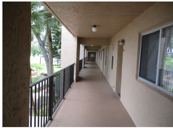
18 2nd Floor Walkway Overview
