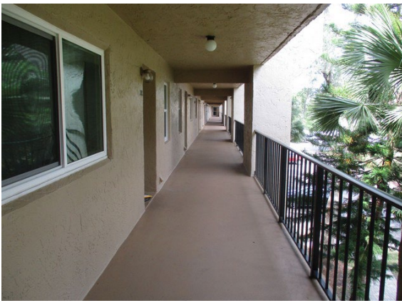
17 3rd Floor Walkway Overview
