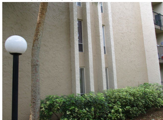
24 Front of Building
