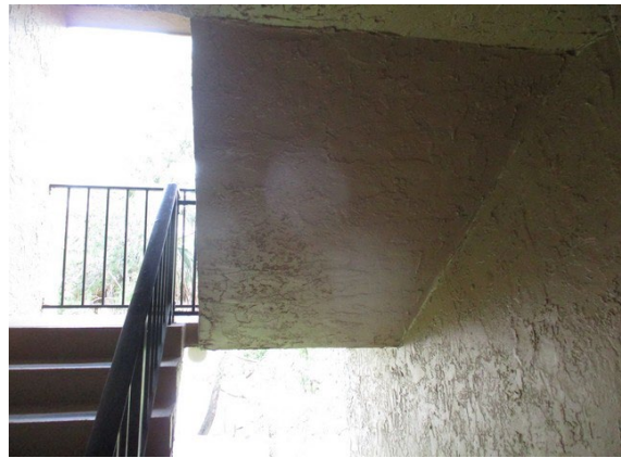
22 Left Stairwell Overview
