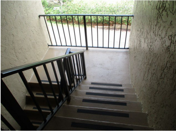
19 Center Stairwell Overview
