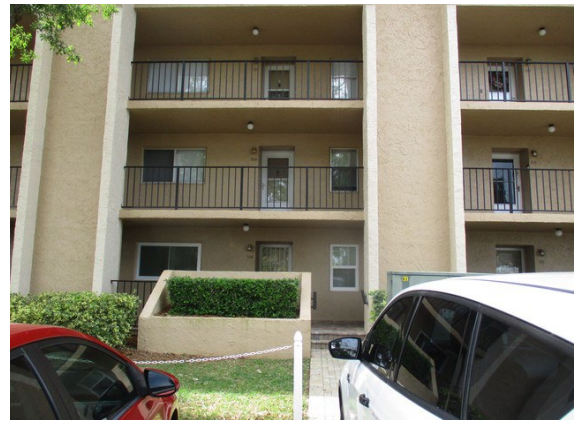
26 Front of Building
