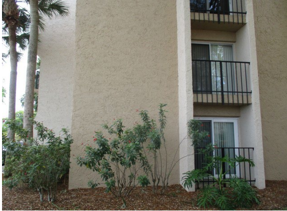
27 Right Side of Building
