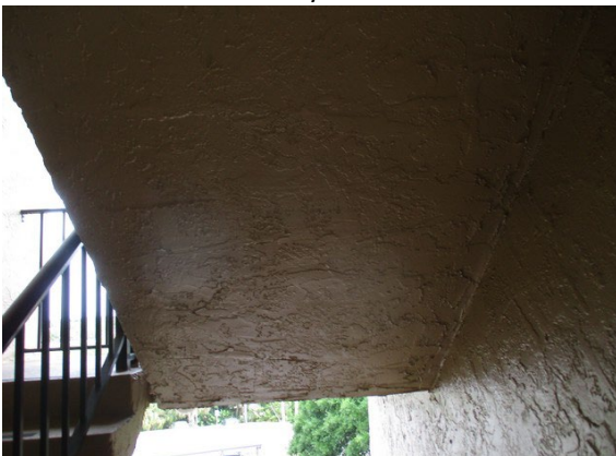
15 Right Stairwell Overview
