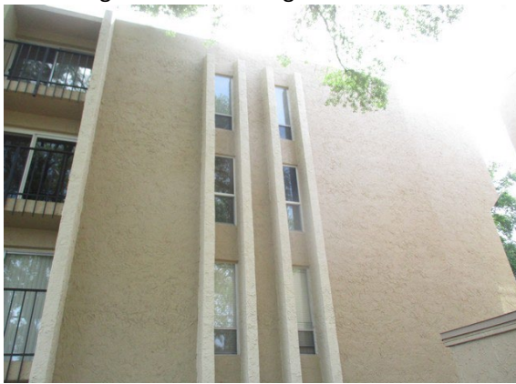
29 Right Side of Building
