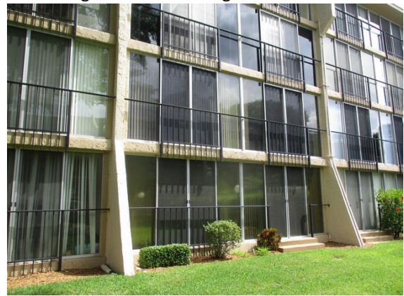
30 Rear of Building
