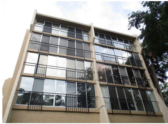
34 Left Side of Building
