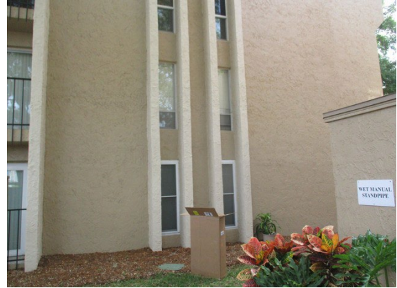
28 Right Side of Building
