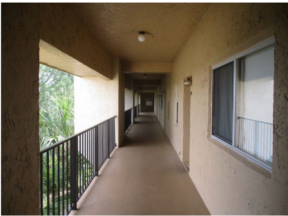
13 4th Floor Walkway Overview
