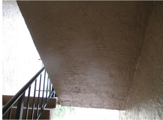
20 Center Stairwell Overview
