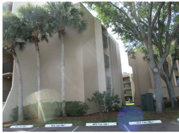
2 Right Side of Building A
