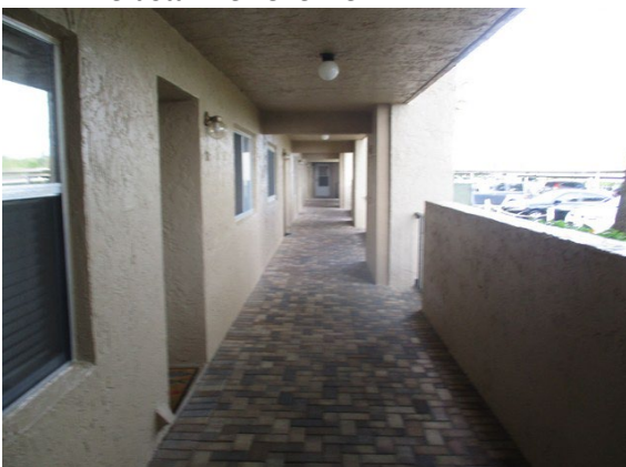
23 1st Floor Walkway Overview
