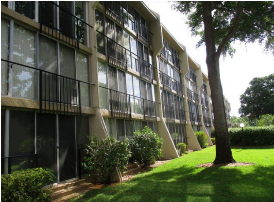
3 Rear of Building A
