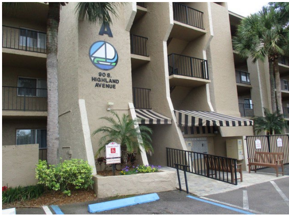
25 Front of Building
