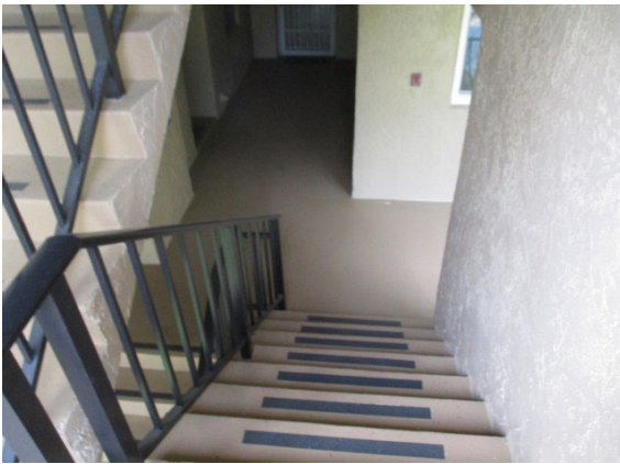
21 Left Stairwell Overview
